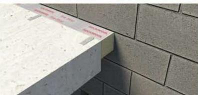
Facade movement must be accommodated by a flexible seal that must be adhered or mechanically fixed to the slab according to the manufacturer's guidelines.
